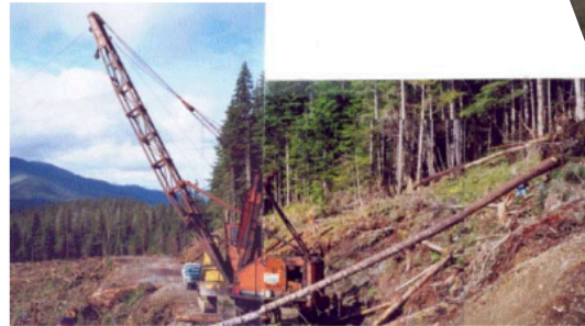
Figure 2. View of swing yarder on access road.
